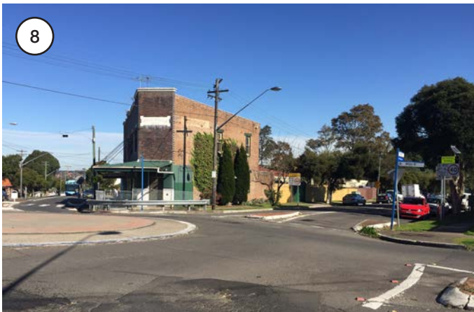
Street condition of Milton and Trevenar Street junction
