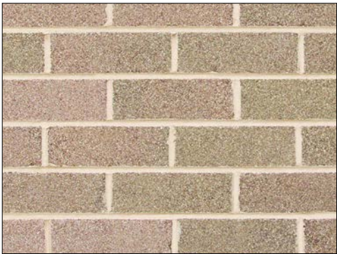
BWK(2) Face Brickwork Type 2 Bowral 76 Simmental Silver or similar
