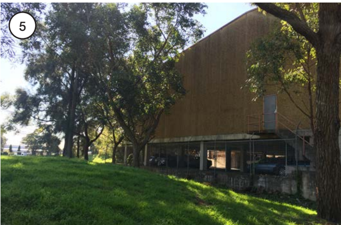
South-western edge condition of site
