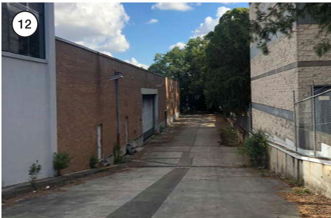
Condition of northern edge of site featuring the existing driveway
